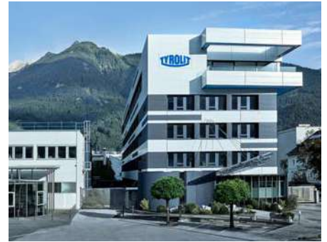
Tyrolit headquarters in Schwaz (Austria)
